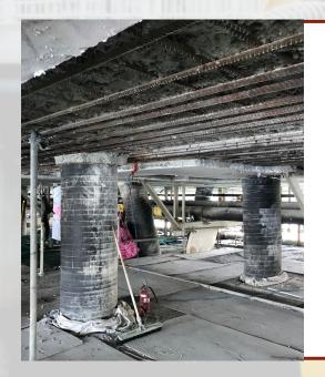
Using our ultra-high-pressure water systems, we specialize in delivering safe and precise hydro demolition and surface removal services for concrete and coatings. Our methods are perfect for exposing rebar, preparing bond surfaces with meticulous control, and effectively eliminating deteriorated or contaminated concrete structures. This technique also minimizes dust and vibration, making it ideal for sensitive environments and structural preservation.
