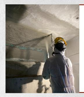
We specialize in applying high-performance shotcrete, both wet and dry mix, for structural rehabilitation and surface protection. Our solutions are ideal for challenging vertical and overhead applications, ensuring long-lasting durability, enhanced load-bearing capacity, and resistance to environmental wear. This method is widely used in infrastructure restoration, tunnels, bridges, and retaining walls.
